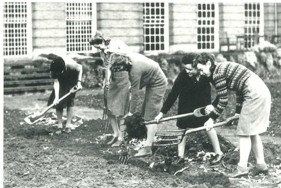
Digging in the war-time gardens
