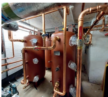
Part of the new air source heat pump system
